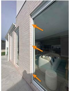
The articulation joint does not extend as the window has been installed tight to the brickwork. The window should have a 10mm gap that is sealed to allow for movement
