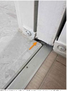
Waterstop should return around the tile under the cavity slider in the laundry
