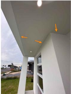
Gaps noted between the ceiling lining and render cladding. Either a trim or sealant should be installed for an adequate finish
