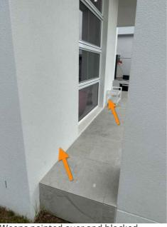
Weeps painted over and blocked. These weep holes have been installed at the incorrect height
