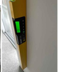
Wall next to backing door is out 6mm over 1200mm
