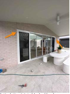
Articulation joints blocked by door system being installed tight to the brickwork
