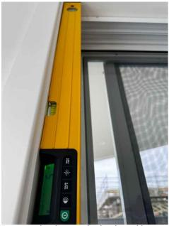
Door set leading to the backyard has been installed out of square
