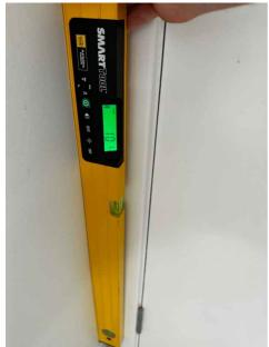
Wall next to external laundry door is out of plumb by 10mm over 1200mm
