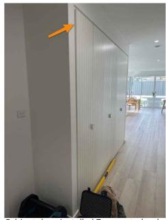
Cabinet door installed 7mm out plumb and does not line up with the wall
