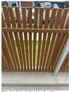
Balustrade installed poorly with uneven gaps common
