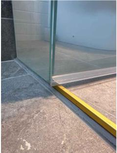
Waterstop angle should extend to the top finished tiled height outside of the shower. The waterstop angle installed only sits 3mm above the finished tiled height in the shower
