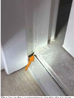
The laundry waterstop angle does not extend the full required length. This is non compliant
