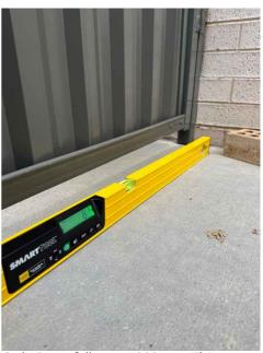
Only 8mm fall over 1200mm. This should be 20mm
