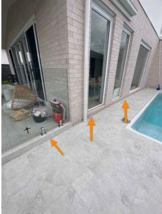
Flexible sealant should be installed to all floor and wall junction areas. This is required to all external areas
