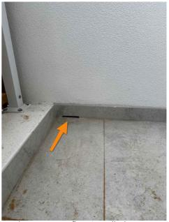
Inadequate overflow installed
