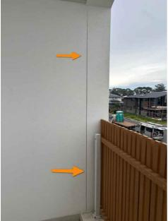
Join between 2 panels requires sealing
