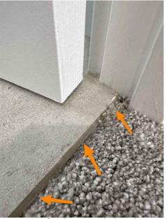
Waterstop finishes 6mm below the finished tiled height in the upstairs bathroom
