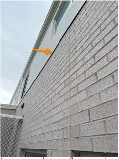
Excessive gap between flashing and brickwork
