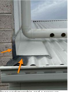
Poor workmanship and a pressure flashing should be installed over the top of this flashing. This is non compliant works
