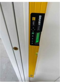
Bow in plasterboard between wall and Laundry cavity slider has been installed out of plumb
